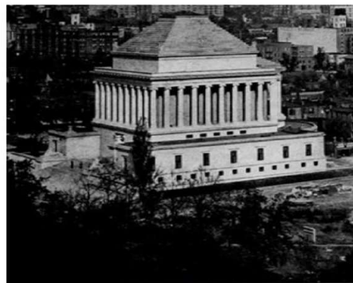
View of Building, Showing Solid Limestone Roof
